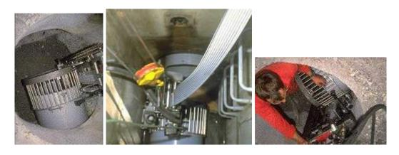
Mechanical matching of strip edges, fixing with comb and rubber seals ensuring water tightness:
