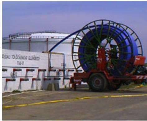
Insertion of the Compact Pipe
