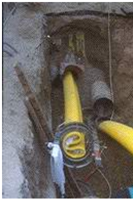
Compact Pipe folded into "C"-shape
