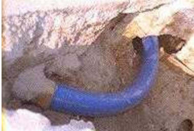
Compact Pipe pulled in an angle
