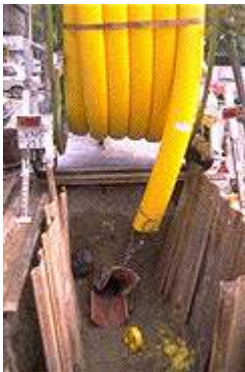
Insertion of the Compact Pipe
