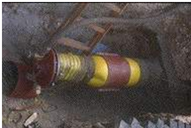
Compact Pipe being inflated
