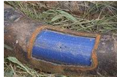
Compact Pipe in the old pipe
