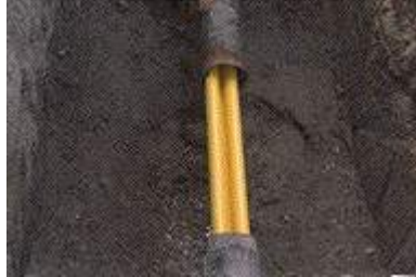
Compact Pipe pulled in
